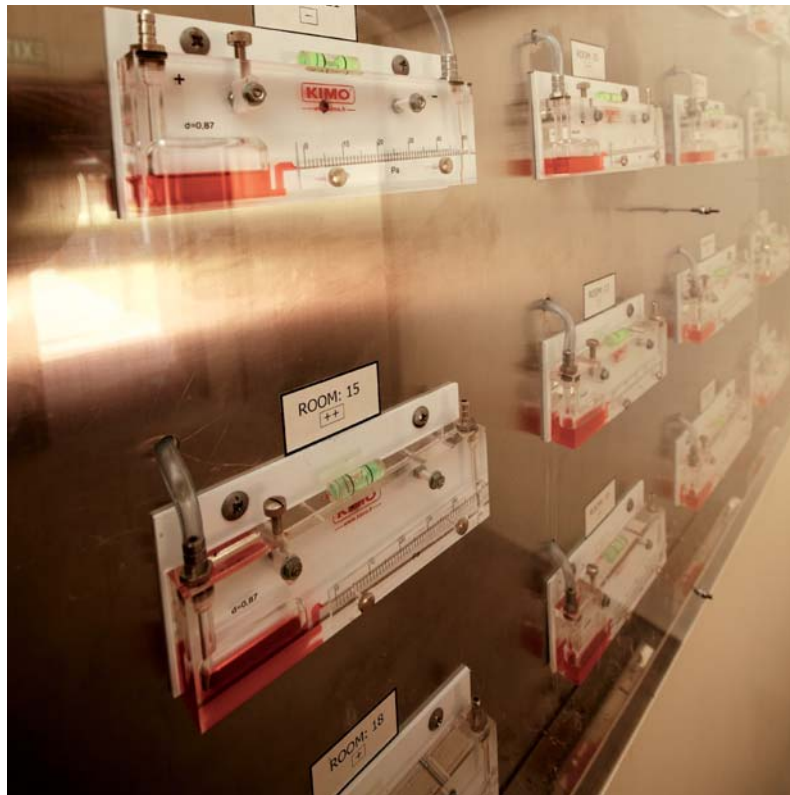
Locked down: the positive room pressure system prevents cross-contamination of operating theatres
